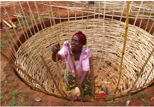
Bamboo-based biogas systems are among the most affordable versions in India and Uganda. a) Traditional weaving skills are a basis for bamboo-reinforced biogas domes and can provide additional income for women; b) Clean gas is led into the kitchen to a gas stove for cooking. Photo credit for the left image: © WECF
